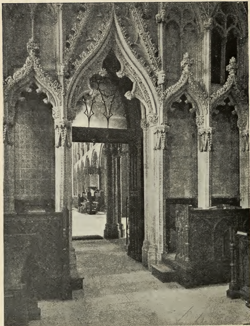
SOUTHWELL CATHEDRAL : THROUGH SCREEN TO NAVE.
